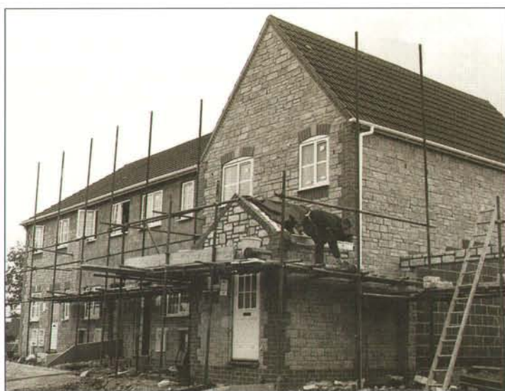
About 50 tonnes of aggregate is required for each new house.
